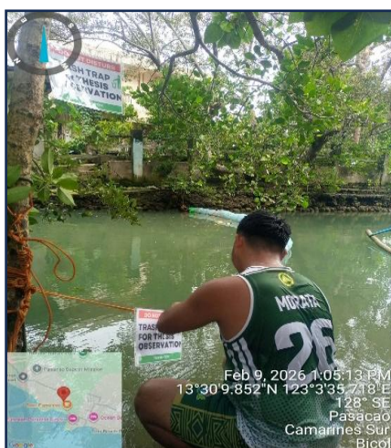
Figure 3. Trash Trap Installation
