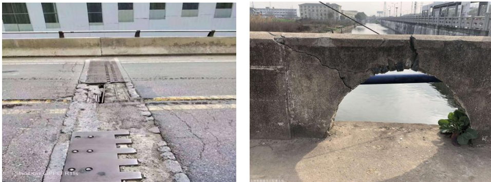
Fig. 2 Diseases of low-grade highway bridges
